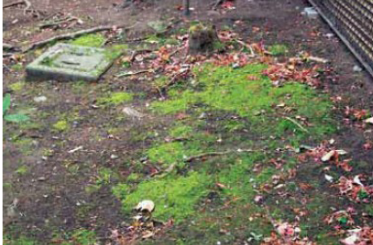
On top of concrete
